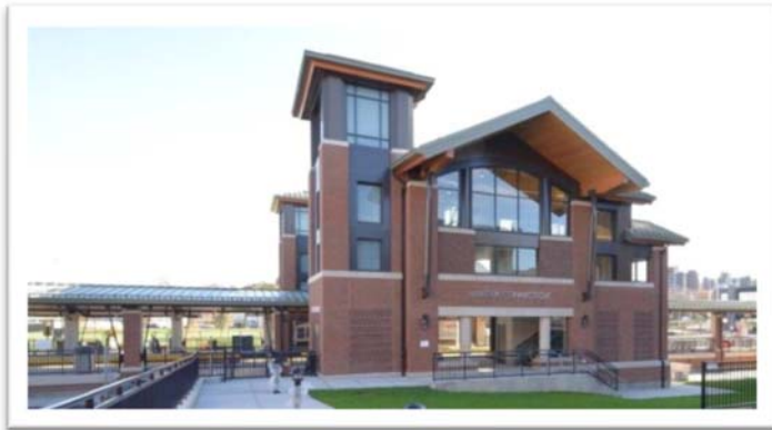
1 Meriden Transit Center
